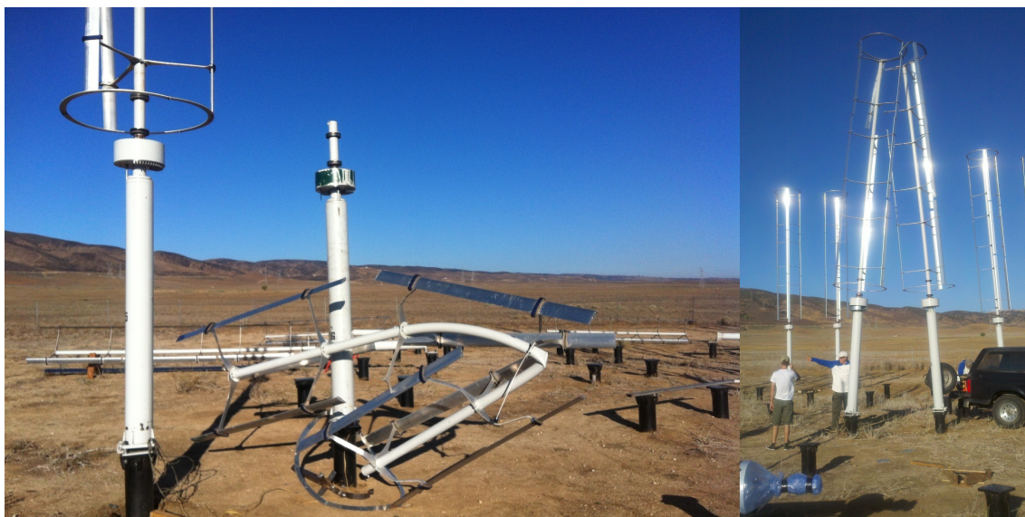
FIGURE 4. Examples of VAWT structural failures at the Caltech Field Laboratory for Optimized Wind Energy (FLOWE).
