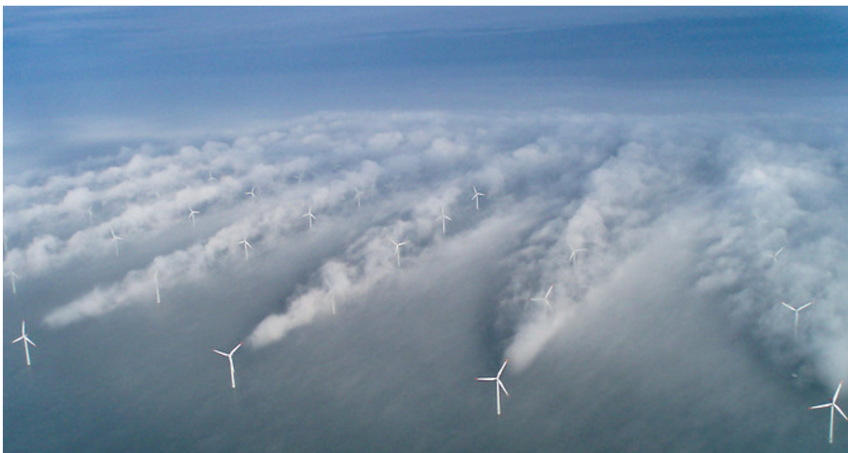
FIGURE 2. Horns Rev Offshore Wind Farm, North Sea. Turbulent wakes visible in fog behind front row of turbines. Photo Credit: Christian Steiness.
